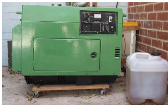
5 kW Diesel generator running on biodiesel
